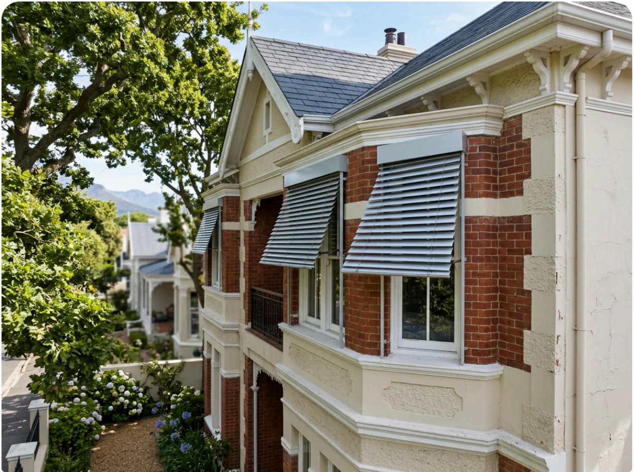
External venetians on the upper storey of a Kenilworth Upper villa — slats turned to hold the view while the direct beam is sent back outside.
